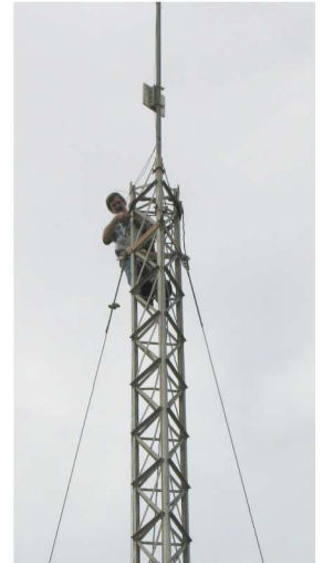
Installing wireless bridge antennas.
