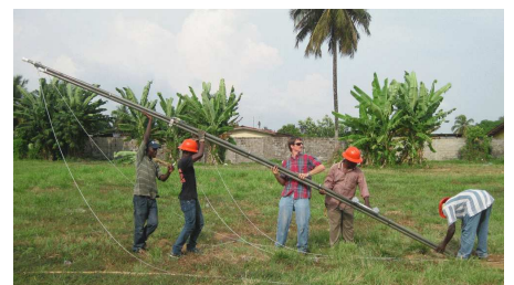
Setting up the new 4.76MHz shortwave antenna, Dec. 2013
