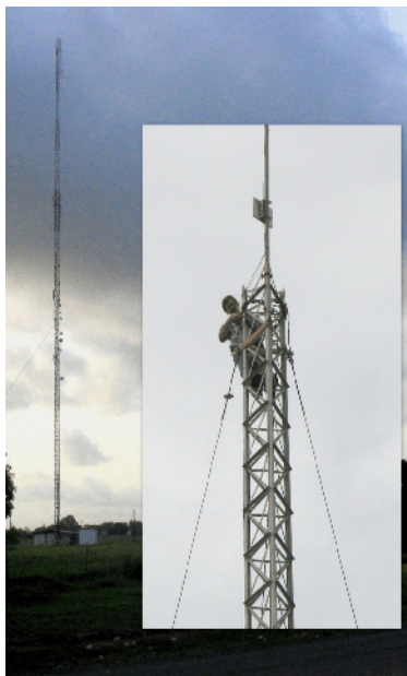
Alan on another ELWA communication tower – he has been getting price quotes on a new 350ft FM tower to replace this one (left), which has a fatal case of “rusting disease”.
